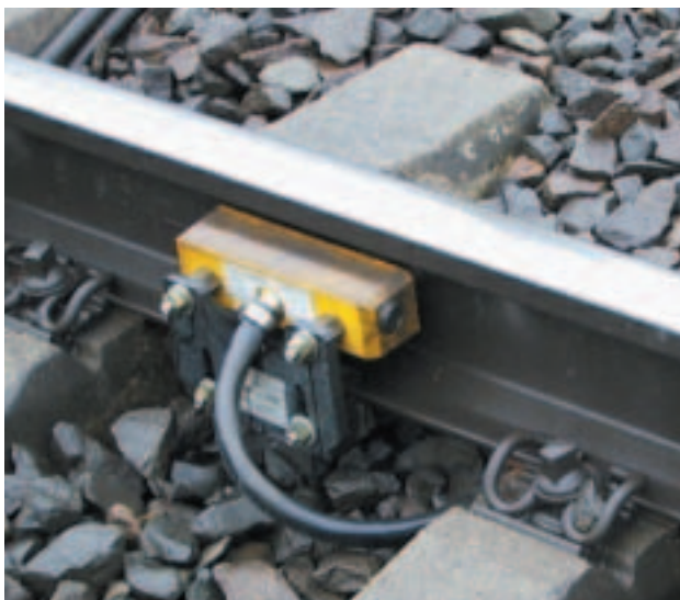
Figure 2: Counting head with wheel sensor RSR122 mounted on rail claw
